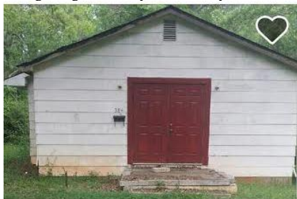
church restoration project
